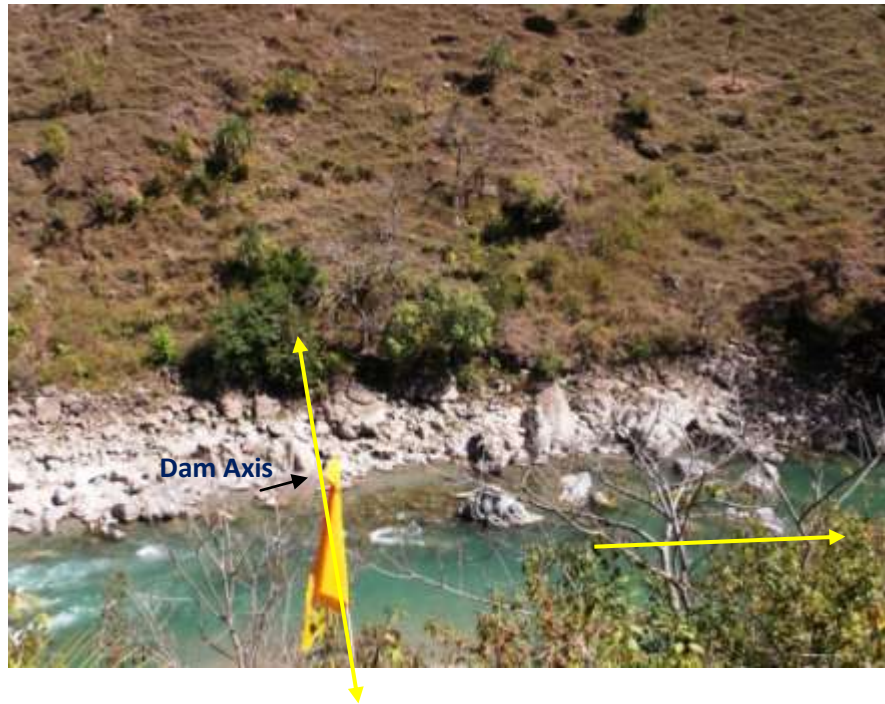
Photo-7: Dam axis into the left bank along flag line.
