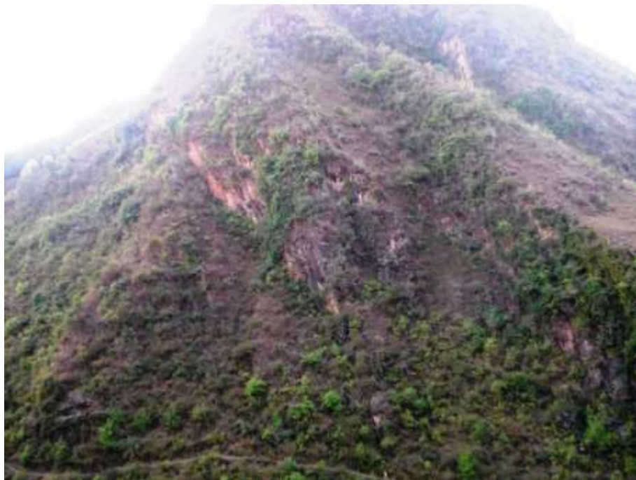
Photo-6: Left abutment uphill near dam axis bedrocks dipping into the hill.
