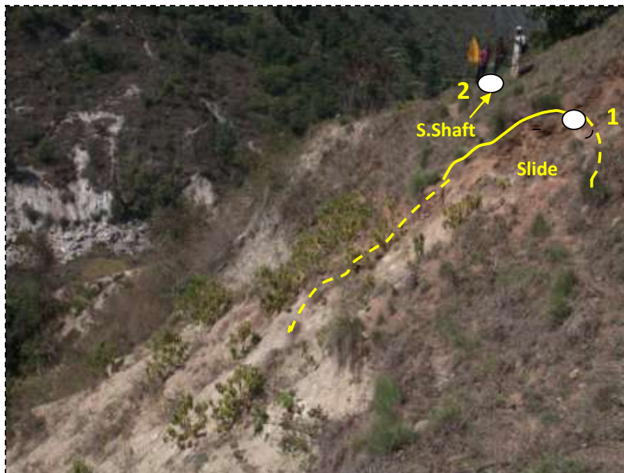
Photo-3. Surge shaft old (1), S. Shaft (2) shifted due to slide.
