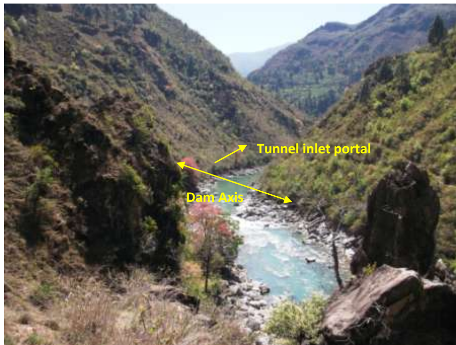
Photo-2: View of Dam axis and HRT inlet portal along left bank of Sarju river course.
