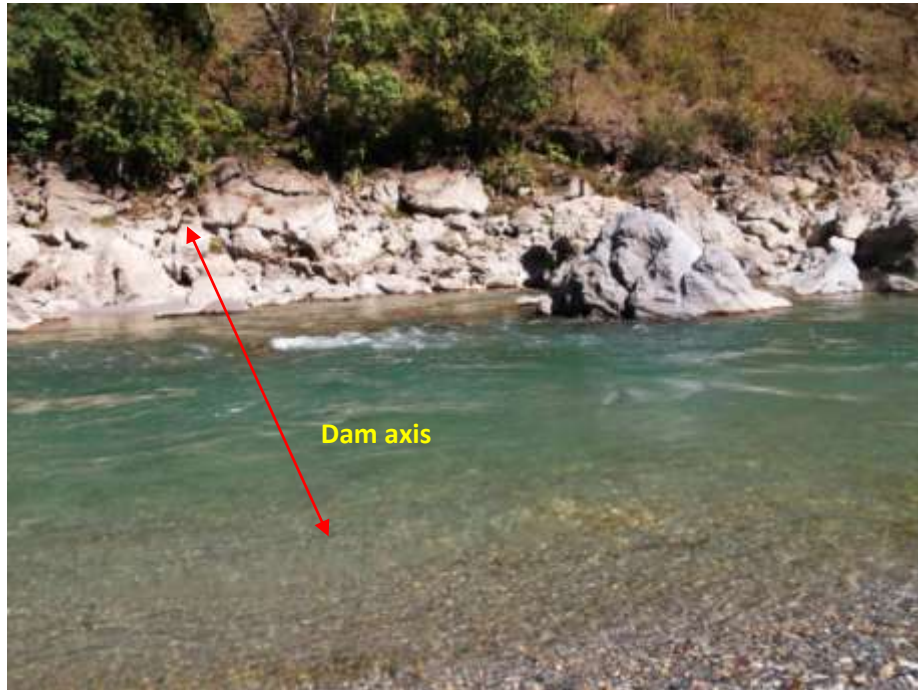
Photo-5: Showing left abutment along dam axis.
