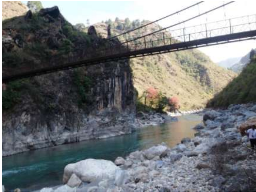
Photo-9: Bedrock at right bank, u/s of dam axis at suspension bridge site.
