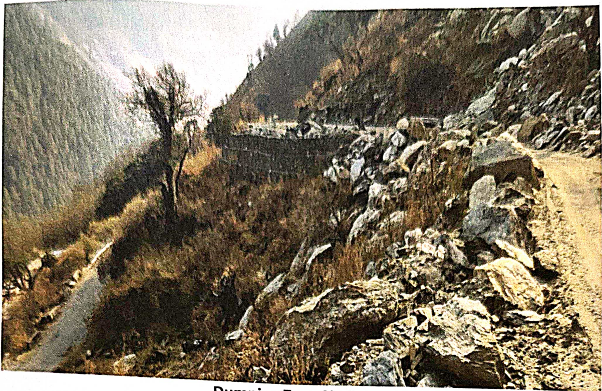
Dumping Zone No-01
