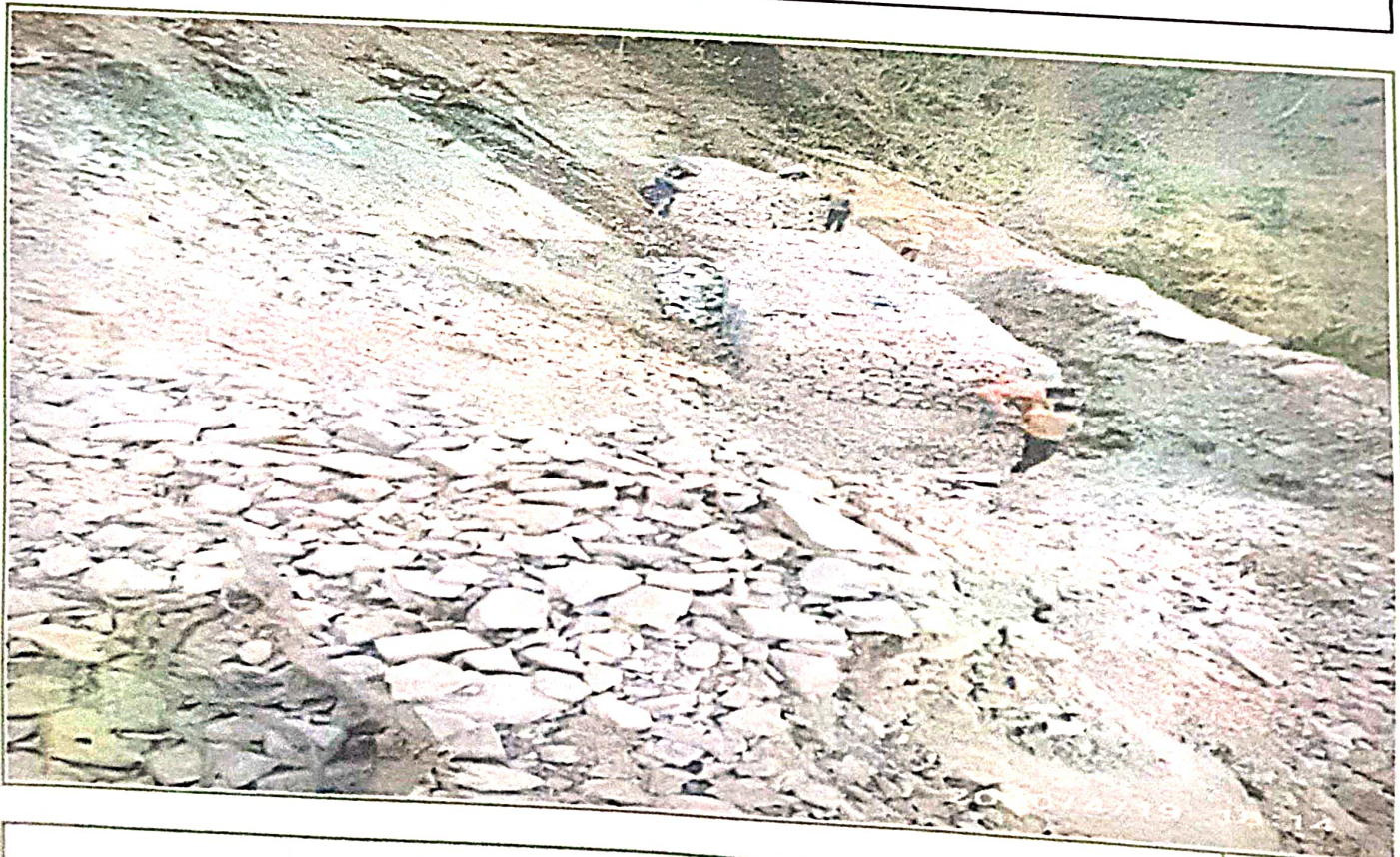
Dumping Zone at Chainge 1.800
