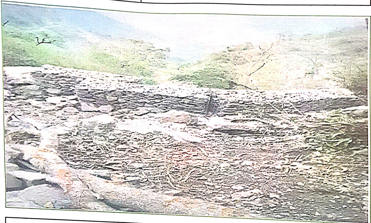
Dumping Zone at Chinage 1.650- 1.750
