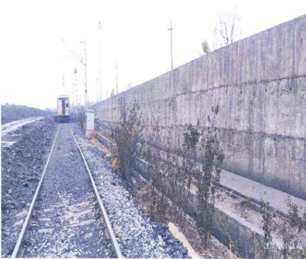
Retaining wall made up of R.C.C of 4m Height have been made on the edge of railway boundary.
