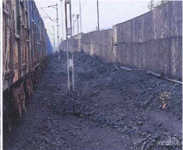
Retaining wall made up of R.C.C of 4m Height have been made on the edge of railway boundary.
