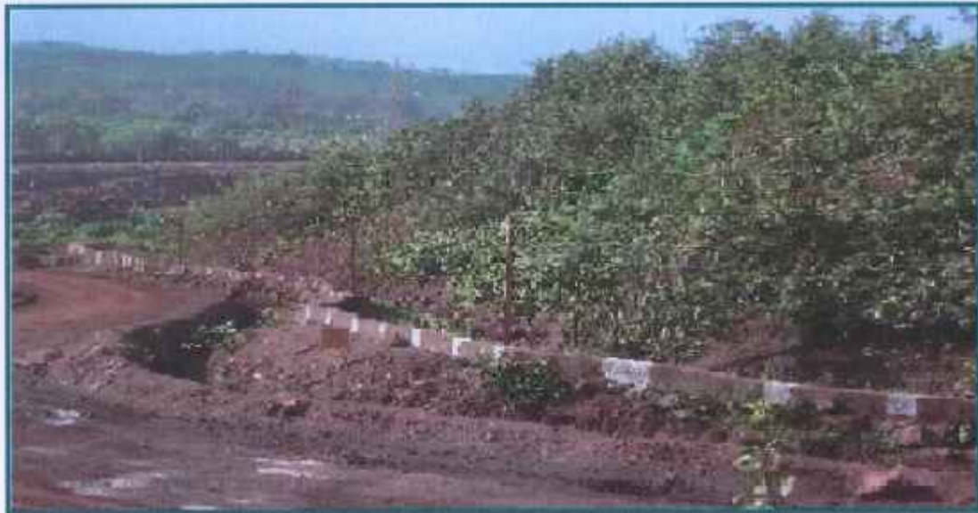
Garland Drain around Waste Dump
