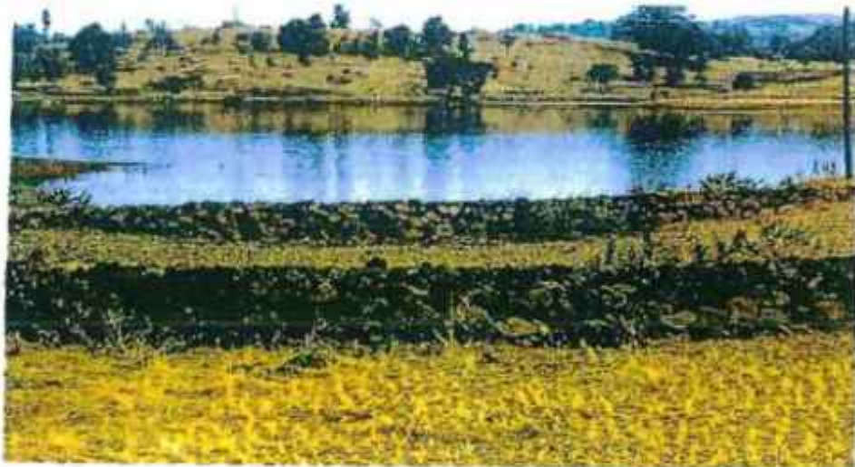
Loose Boulder Structures
