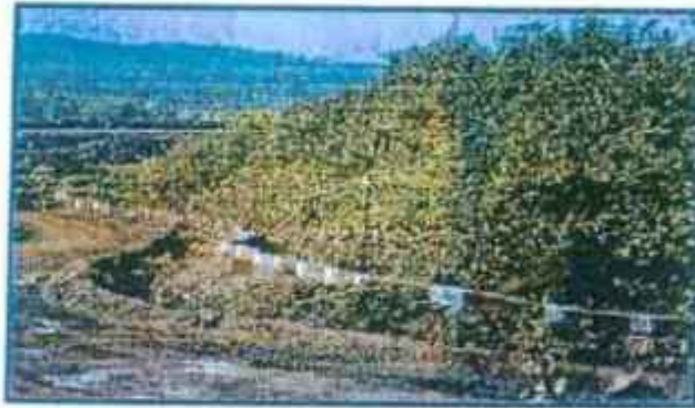
Garland Drain around Waste Dump
