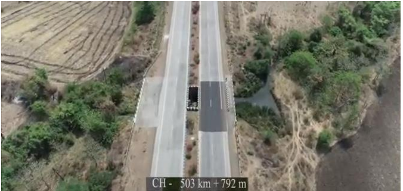
MNB at Km 503.867
