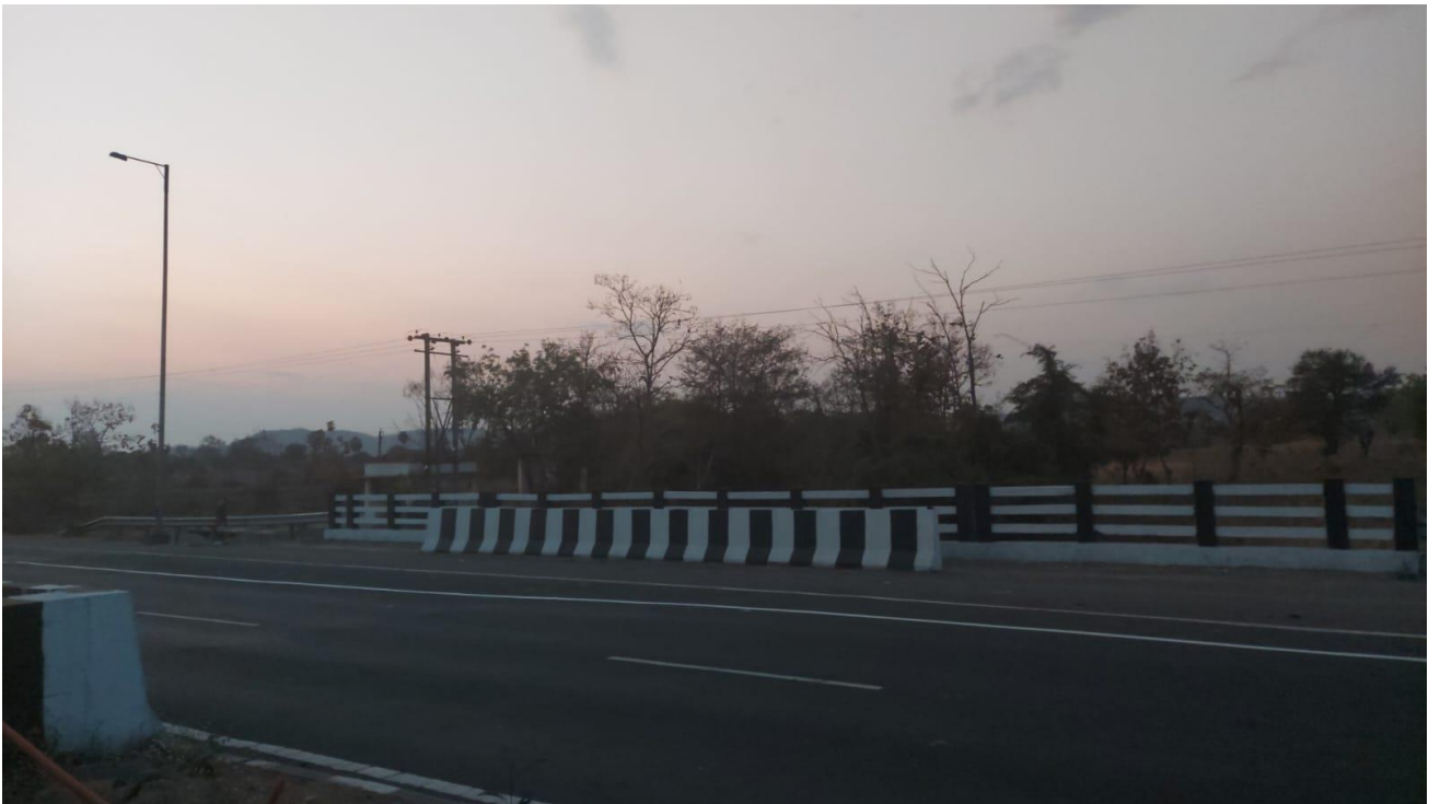
MNB at Km 506.316
