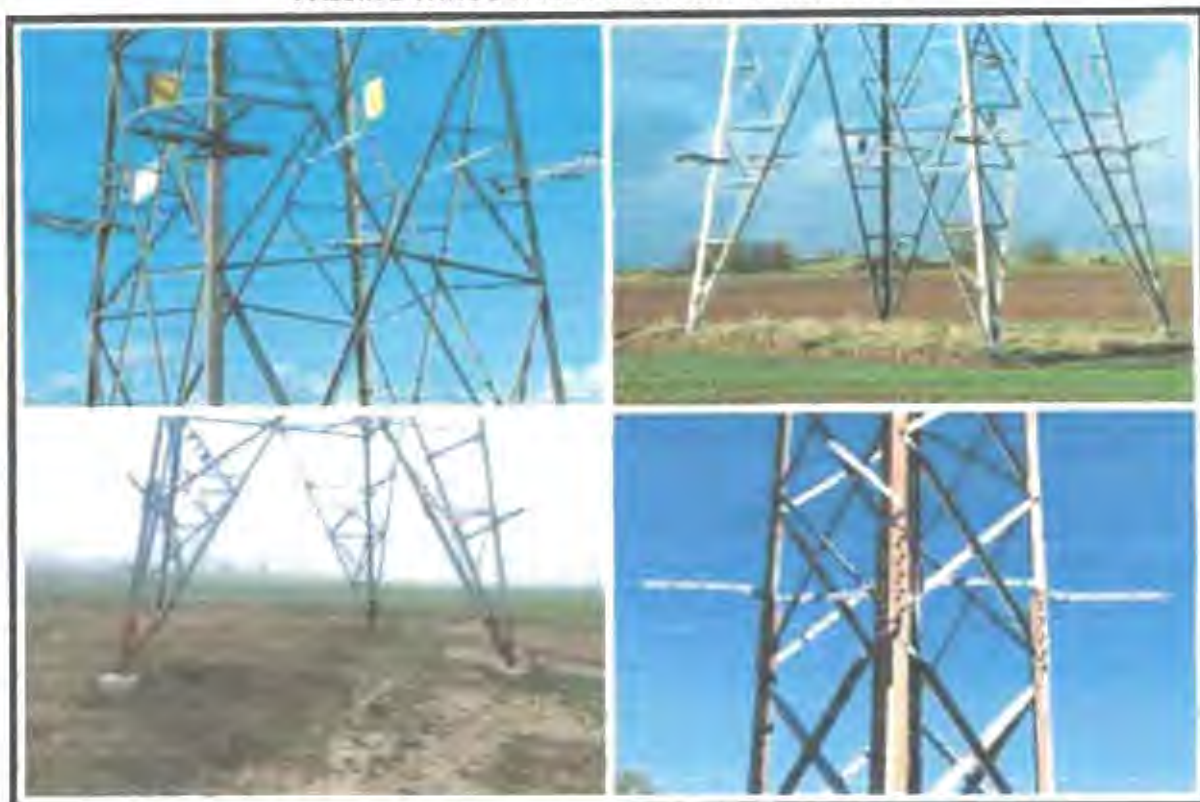
FIGURE 4.C.3: ANTI-CLIMBING DEVICES PROPOSED TO BE INSTALLED ON TRANSMISSION LINE PASSING THROUGH SELECTED FOREST STRETCH
