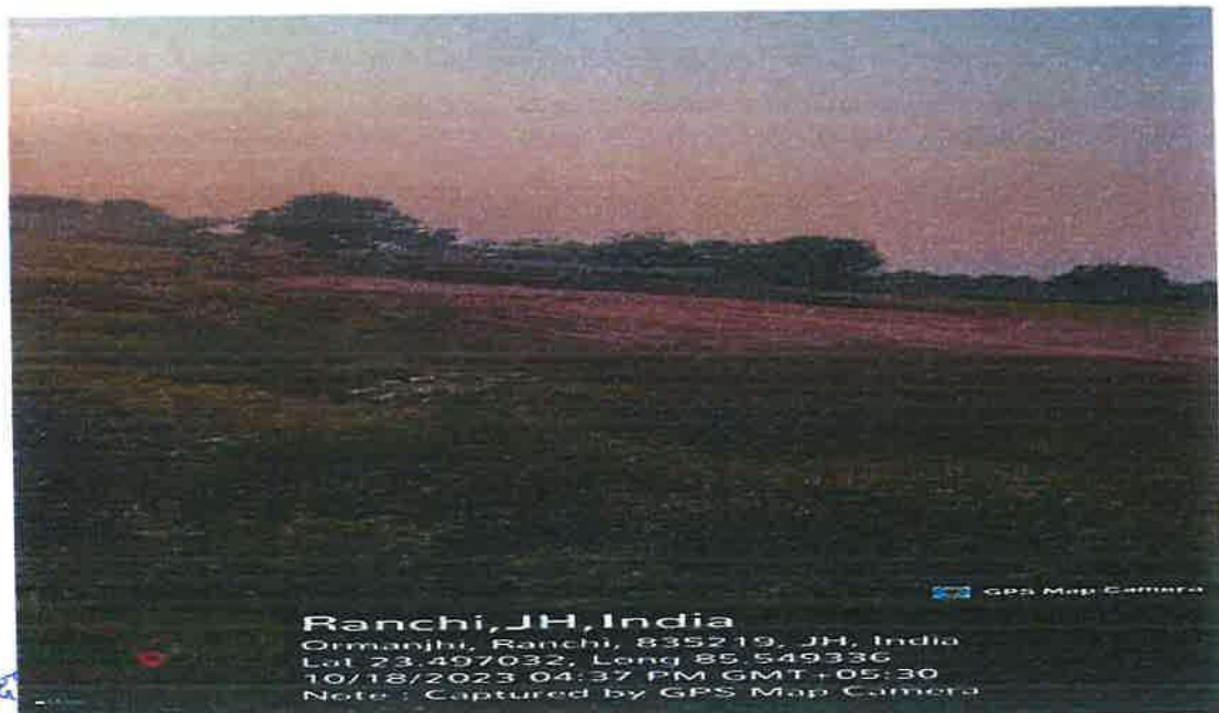
Filling Section Ch75+750
