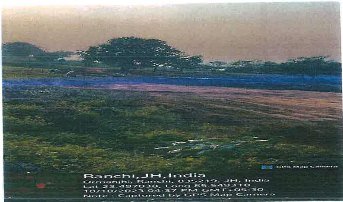
Filling Section Ch75+850
