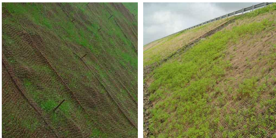
Example of Geotextile Mats
