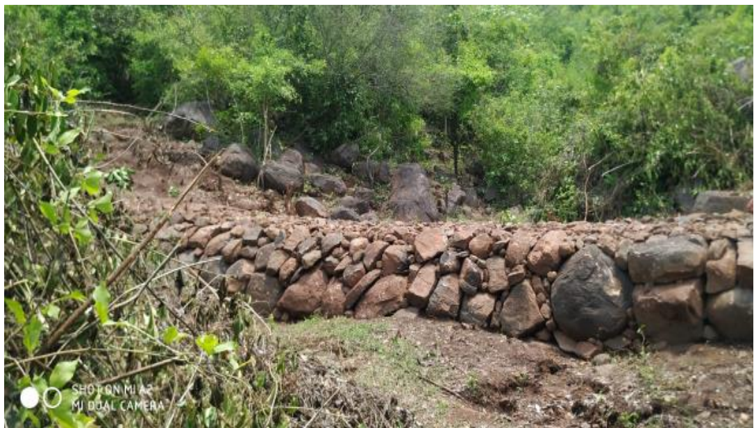
Construction of Loose Boulder Structure
