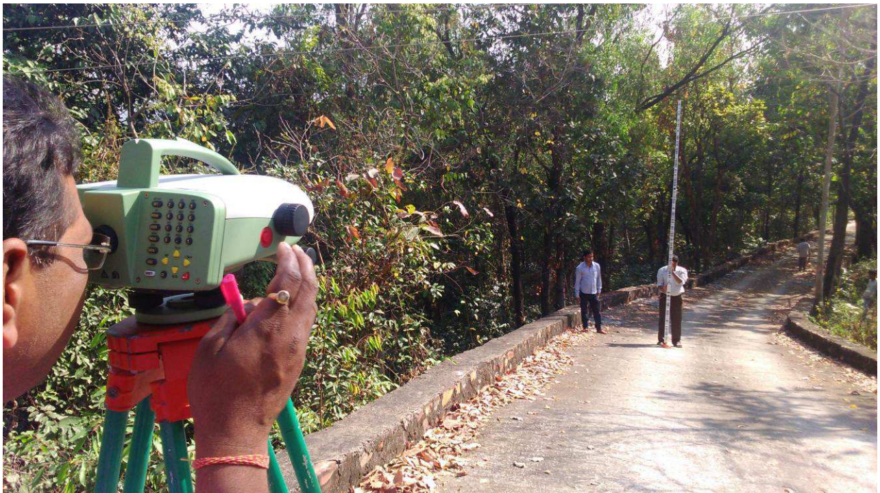
Fig. 13b: Monitoring of elevations at subsidence monitoring stations using precise digital level
