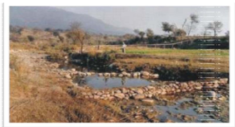
Drain line treatment with stone wall.
