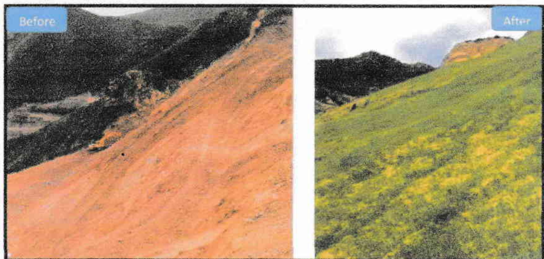
Rehabilitation of slopes using bio-engineering techniques
