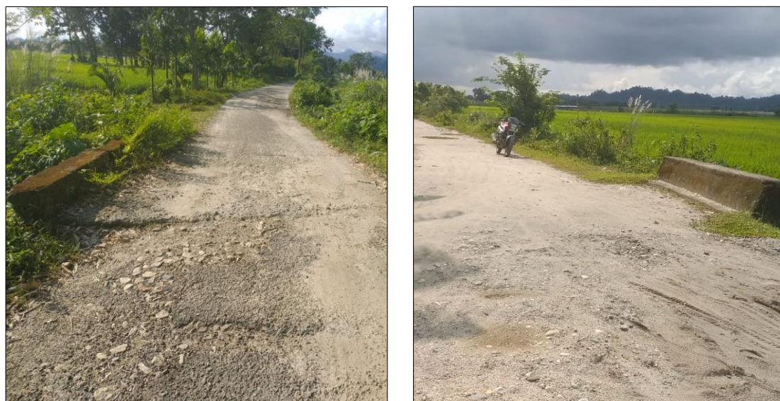
Figure 2-7: Photo of Highly Distressed Road along the stretch
