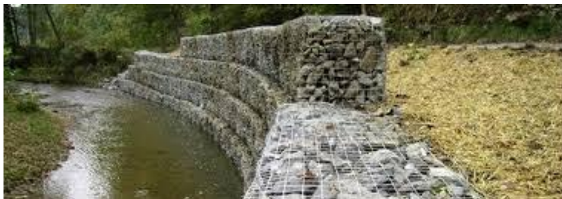
Figure 7-8: Gabion Walls
