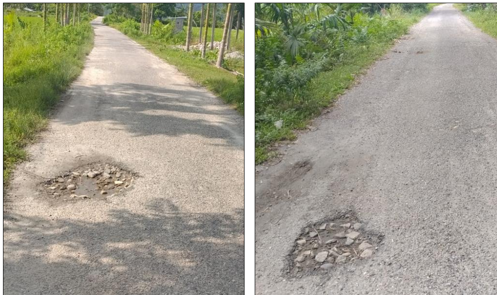
Figure 5-3: Potholes along Project Road
