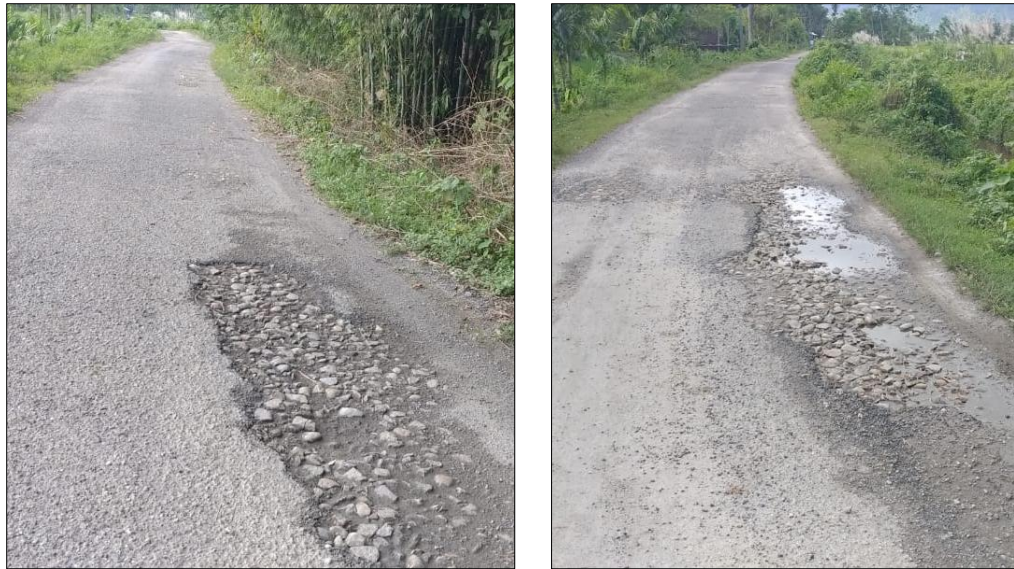
Figure 5-4: Edge Failure along Project Road
