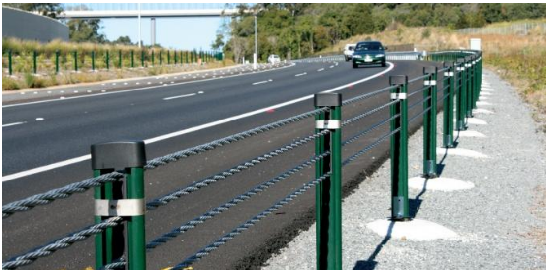
Figure 7-6: Wire Rope Crash Barrier
