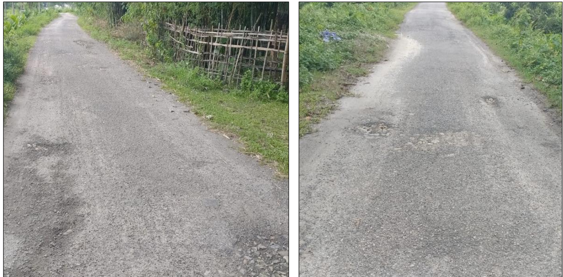
Figure 5-2: Raveling along Project Road
