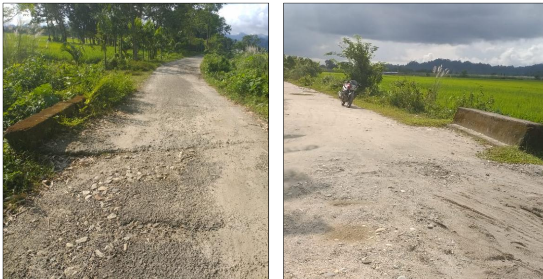
Figure 5-5: Photo of Highly Distressed Road along the stretch
