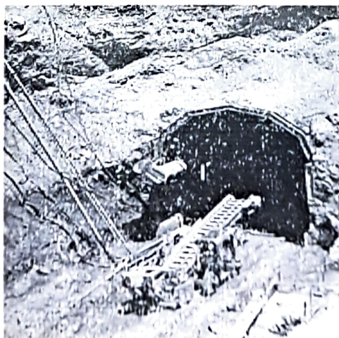
HAGGLUND LOADER MOVING INTO TUNNEL
