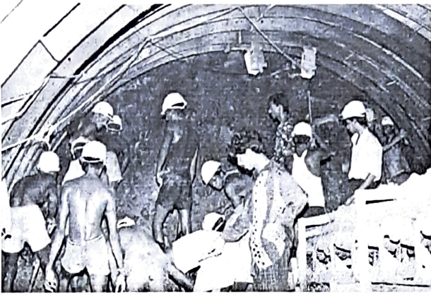
HEADING WORK IN PROGRESS
