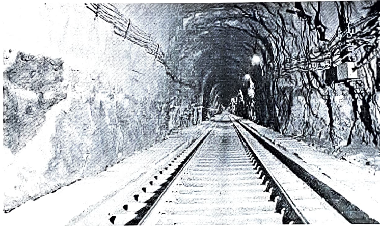
BALLASTLESS TRACK IN KARBUDE TUNNEL
