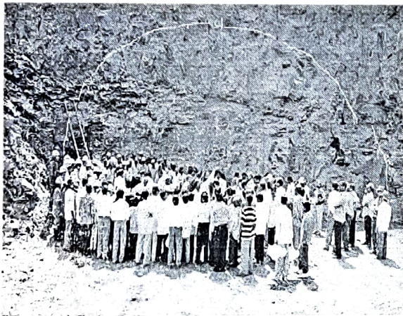
PROFILE MARKING FOR INTIAL BLAST
