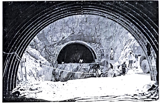
HEADING WORK IN PROGRESS
