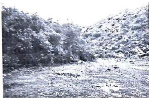
Grassing at OB dump of Kuya Colliery
