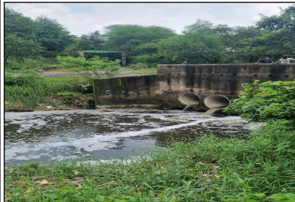
Check dam over Chatkari Jore near Govardhan Eco-park
