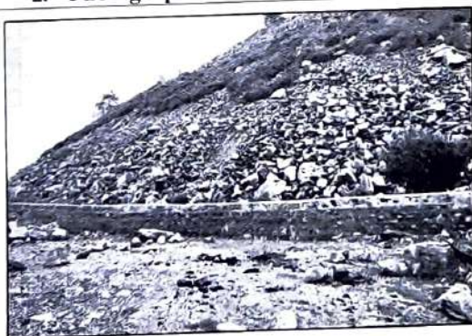
Retention/ Toe wall around OB dump of Bera Colliery
