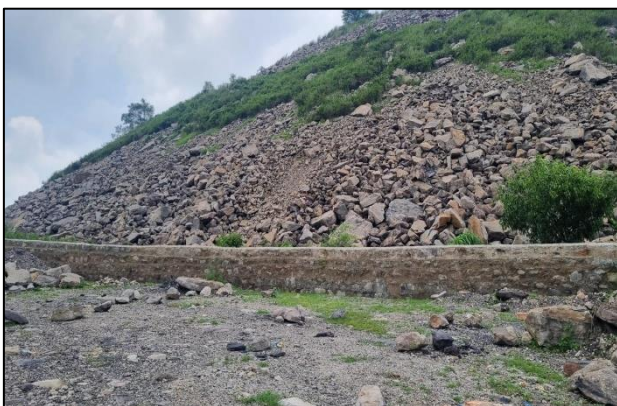
Retention/ Toe wall around OB dump of Bera Colliery
