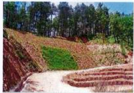
Slope Protection using Bio engineering techniques
