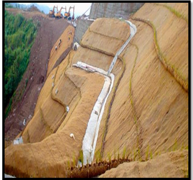
Use of Geo- mats for Slope Stabilization
