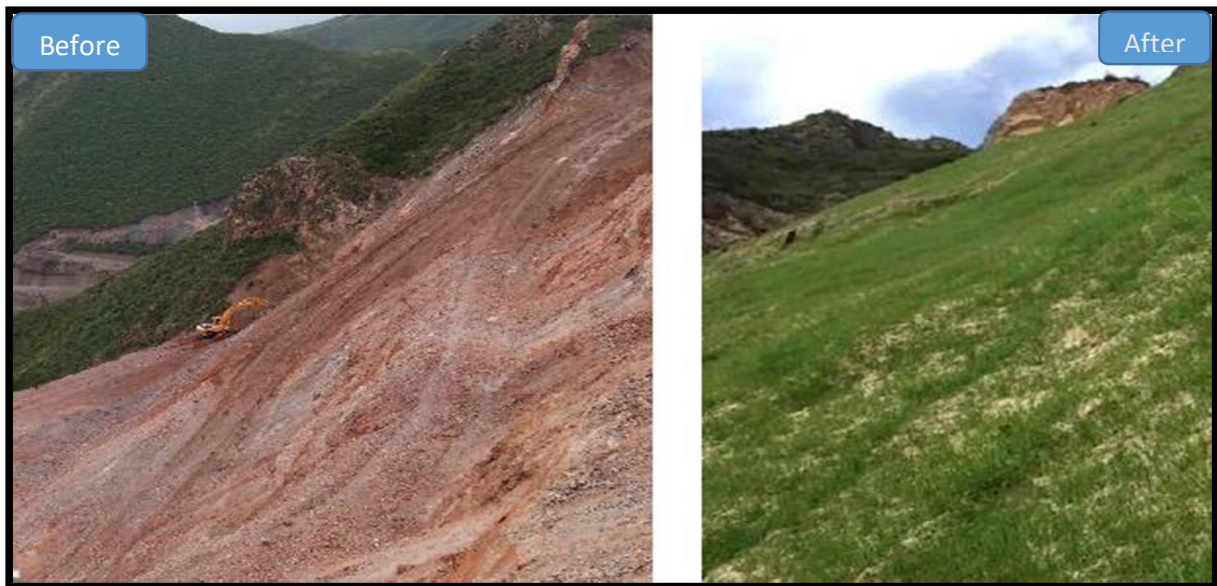
Rehabilitation of slopes using bio-engineering techniques
