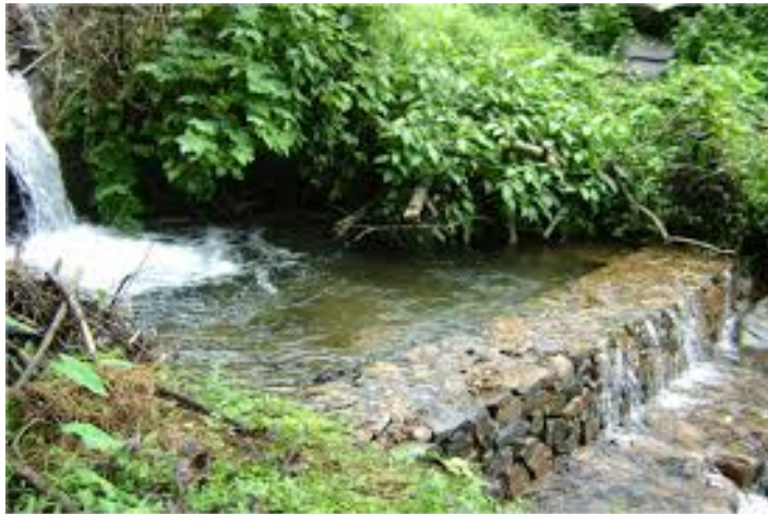
A View of Dry Rubble Stone Masonry Check Dam
