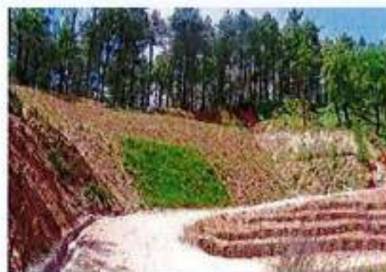
Slope Protection using Bio engineering techniques
