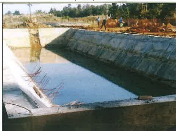
Permanent Settling Tank - 1 nos. 300 m3 capacity
