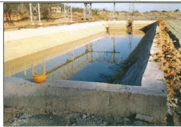
Permanent Settling Tank - 2 nos. of 1800 m3 capacity each
