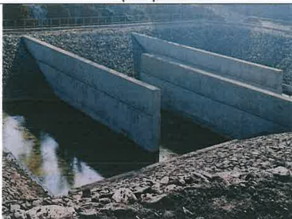
Permanent Settling Tank - 1 nos. 2625 m3 capacity
