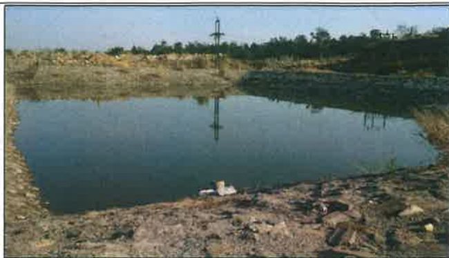
Permanent Settling cum Recharge Tank within Project Area (4000 m3 capacity)
