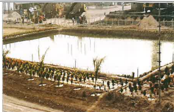
Settling cum Recharge Tank near workshop Area (2000 m3 capacity)
