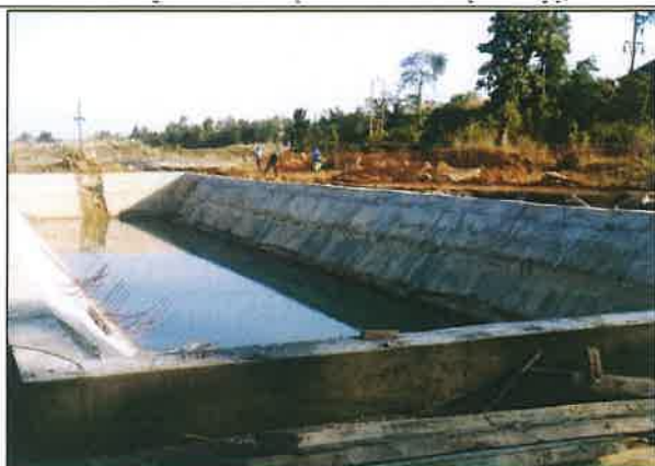
Permanent Settling Tank - 2 nos. of 1200 m3 capacity each
