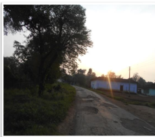
Photo : Ravelling at km CH- 14+000
