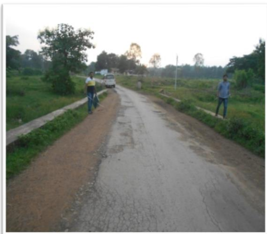
Photo : Map Cracking at CH – 21+000
