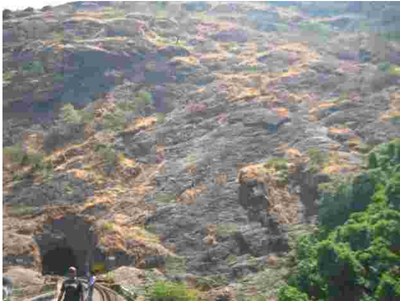
View of Tunnel No.6 in Granite formation
