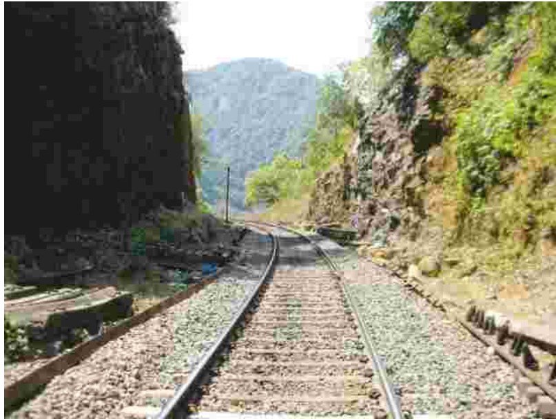
View of cutting in Diorite formation on both sides after Tunnel No. 4
