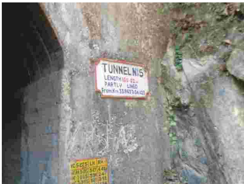
Tunnel no. 5 in weathered Diorite formation
