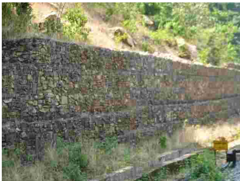
A View of the Gabion structure after station 2 for a stability of weak formation
