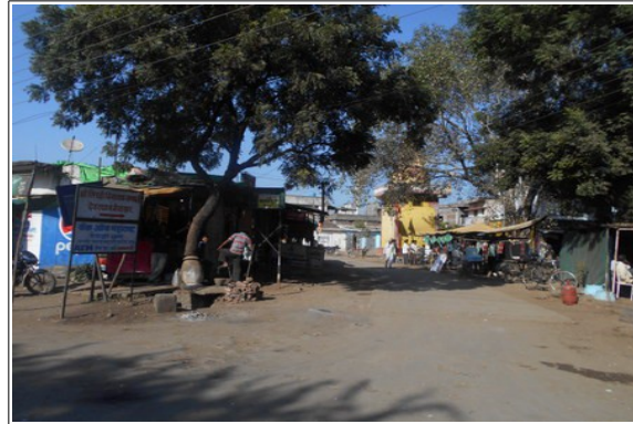
Fig 9.9.4: - Encroached Existing RoW
