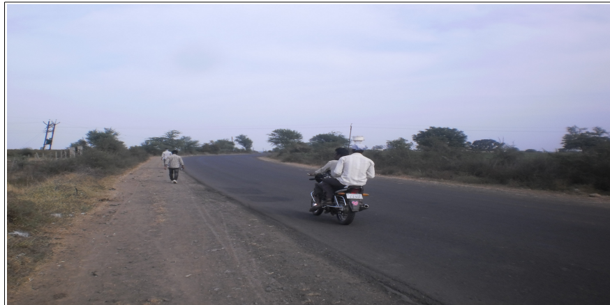
Fig-9.9.1(a): Two Lane Carriageway with Earthen Shoulders
