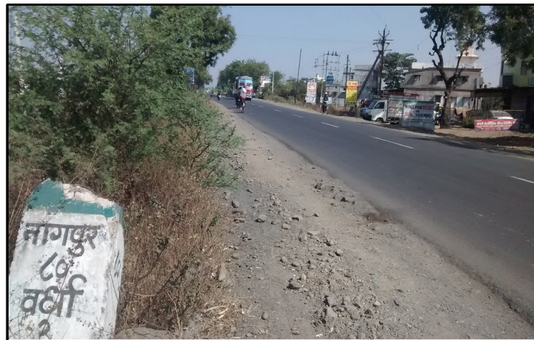
Fig. 9.11.1: Structures are noticed within RoW
