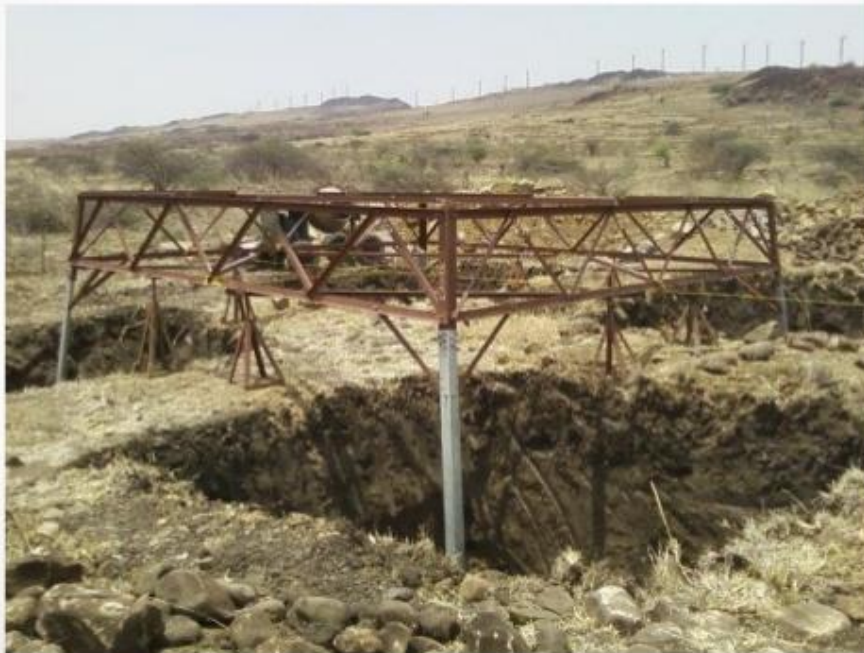
Stub setting & Template Assembly
