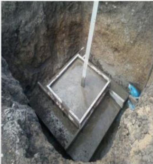
Stub Footing concrete
