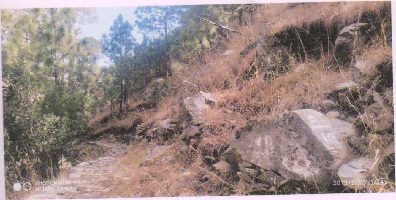
Muck Dumping Yard - C
