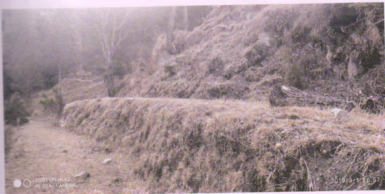
Muck Dumping Yard - I
