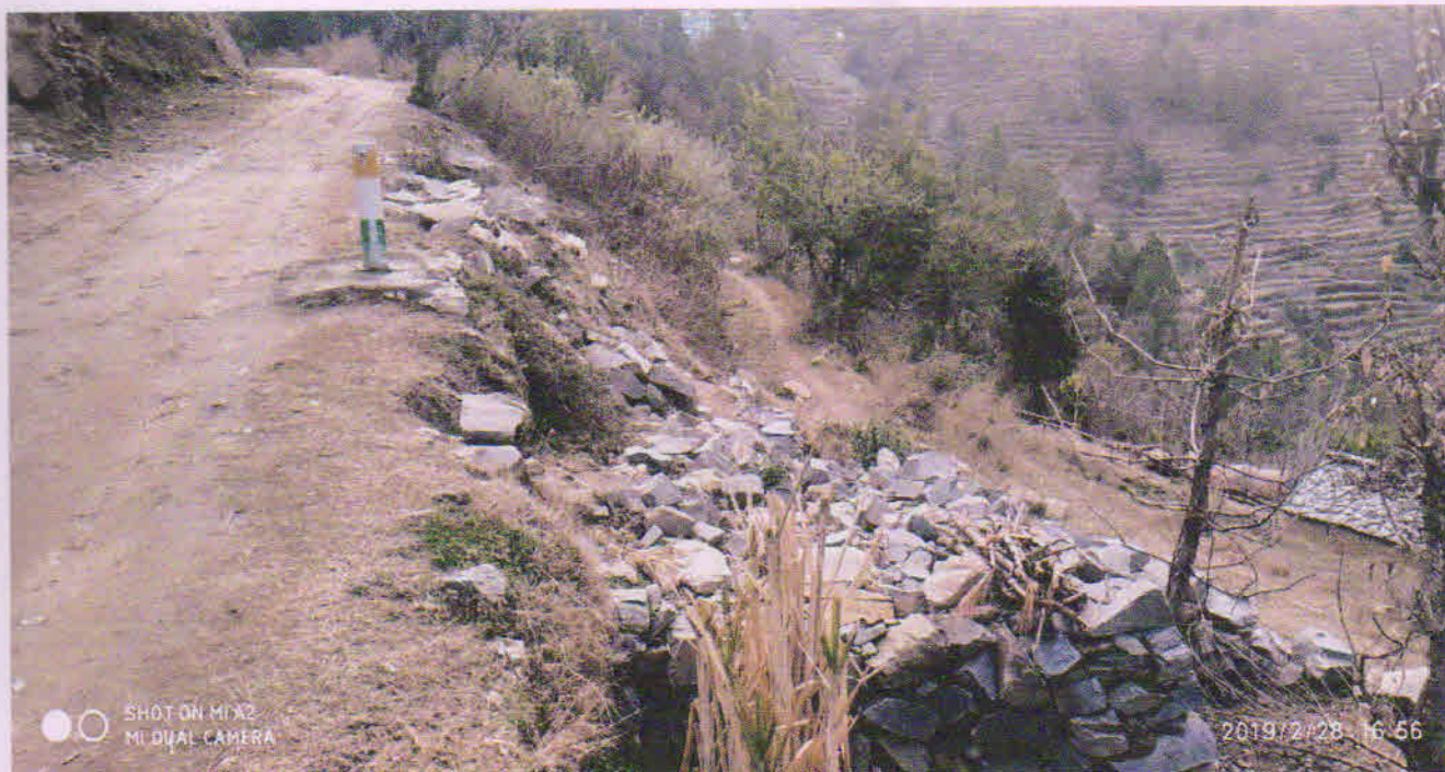
Muck Dumping Yard - A
