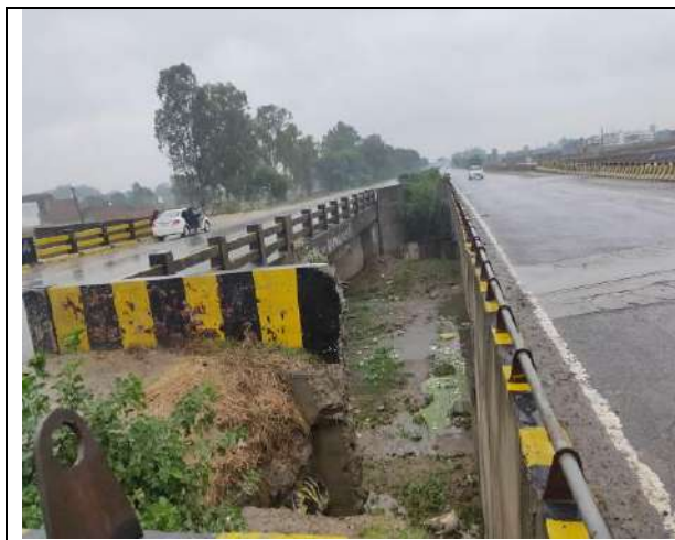
Minor Bridge at Ch. 399+965
