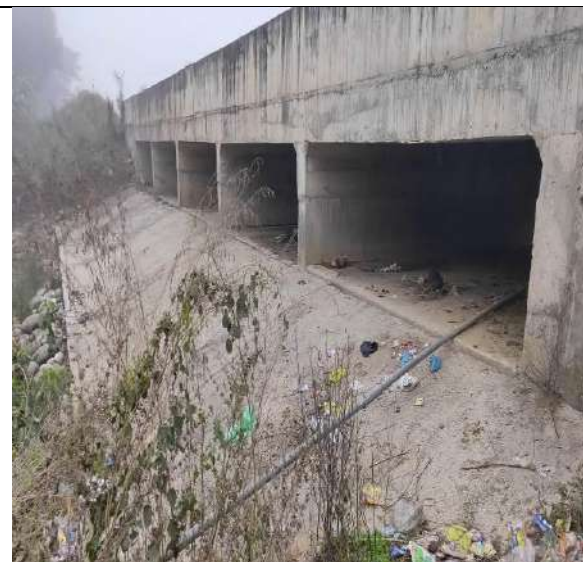
Minor Bridge at Ch. 456+679
