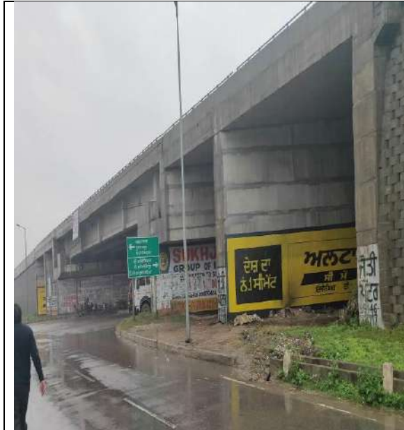
Flyover at Ch. 398+135
