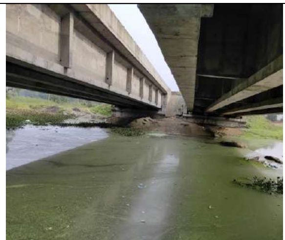
Minor Bridge at Ch. 411+575
