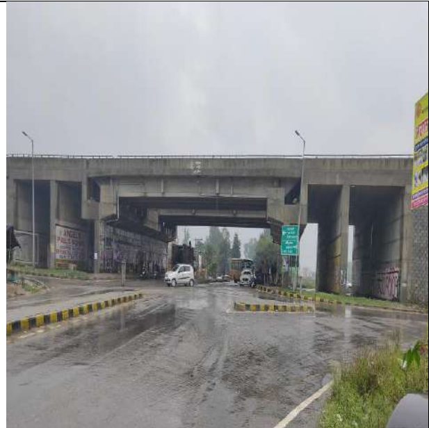
Flyover at Ch. 399+610
