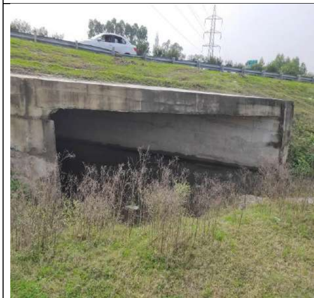
Minor Bridge at Ch. 414+942
