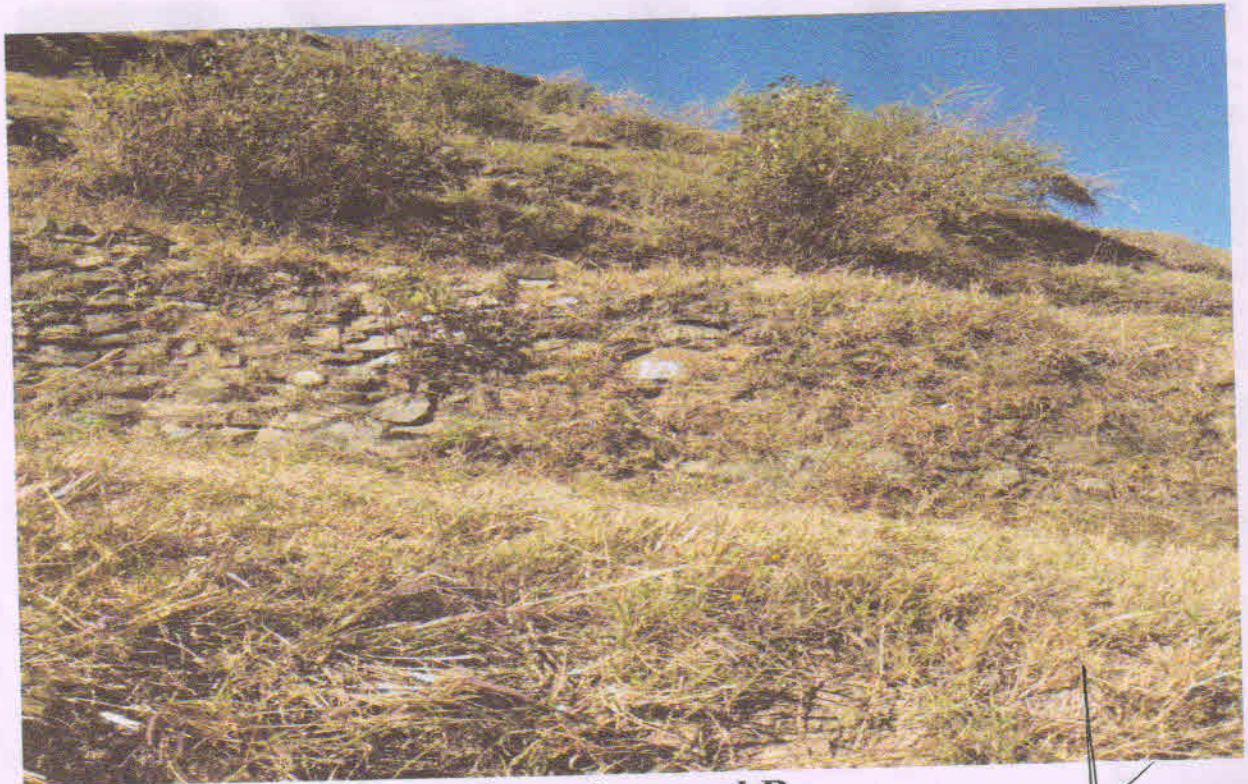
Dumping yard B
