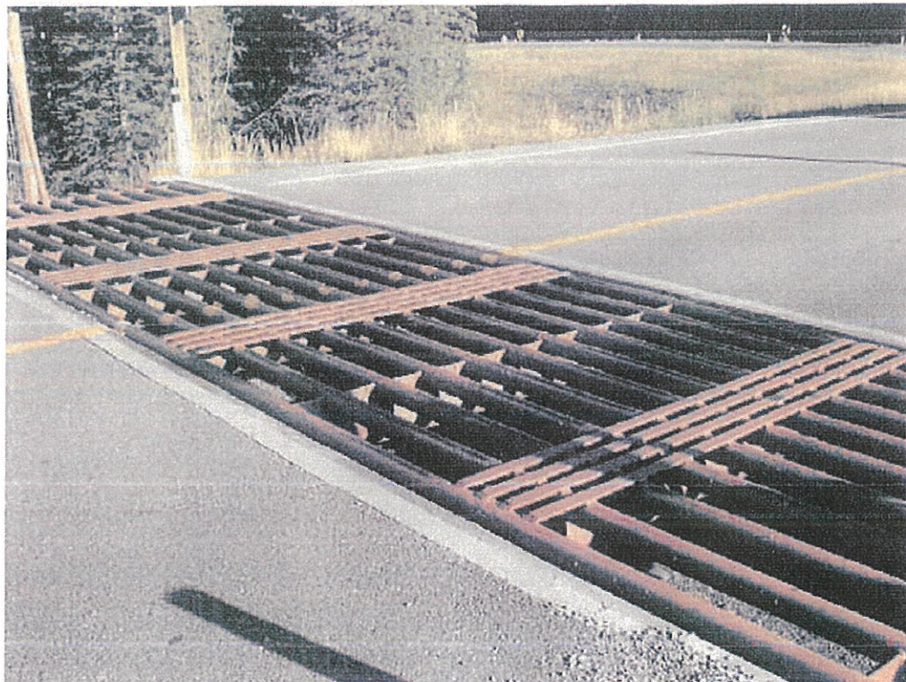
Figure 7: Cattle guards/grids to be installed at both ends of the crossing structure on NH 119 at Chainage 60/350 and 61/050. Source: (Clevenger & Huijser 2011)
