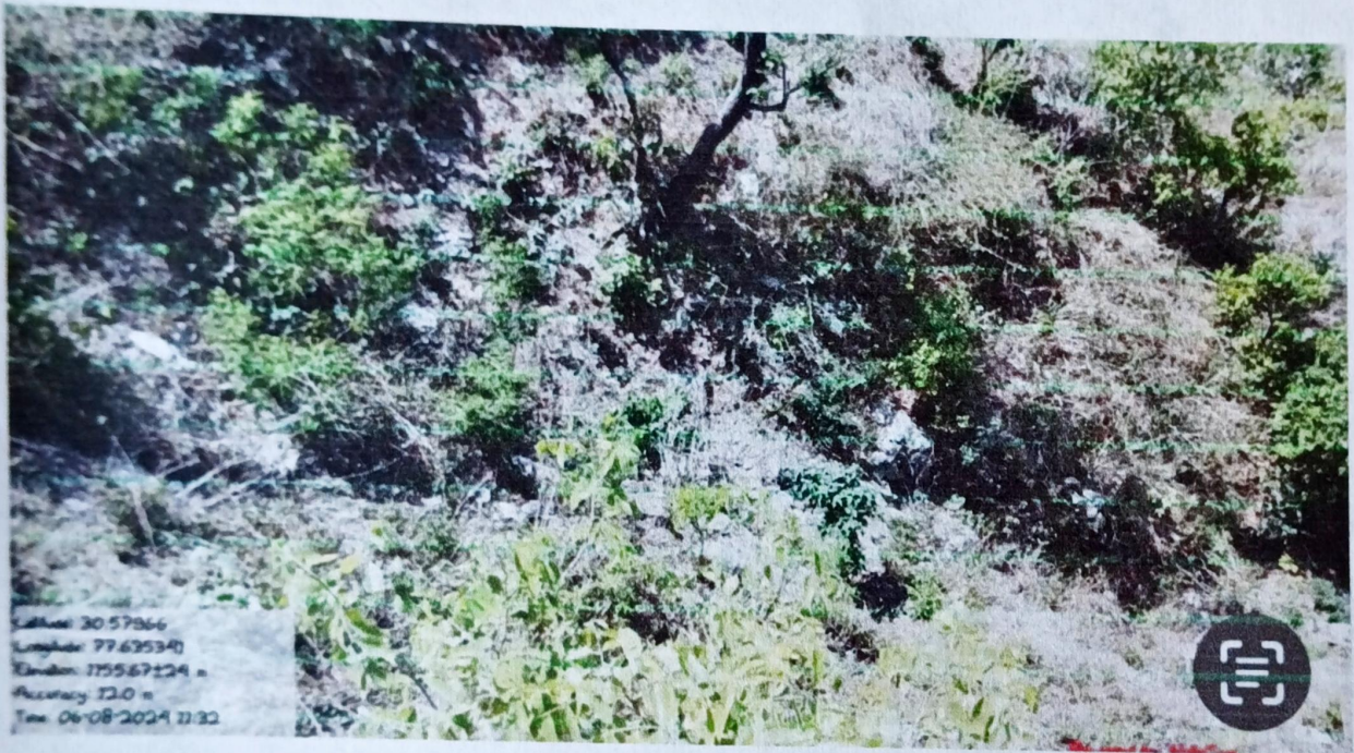
Dumping Site No.4 at RD 3/780 KM
