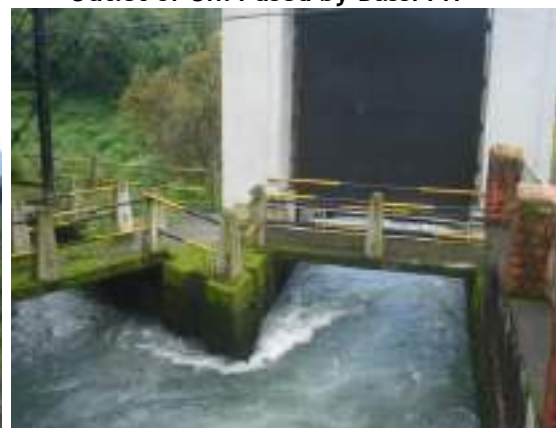
Outlet of Uhl I HEP with open trench
