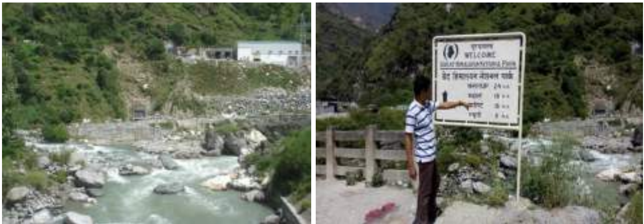
Confluence of Sainj Khad and Jiwa Nala and Power House site of Sainj HEP
