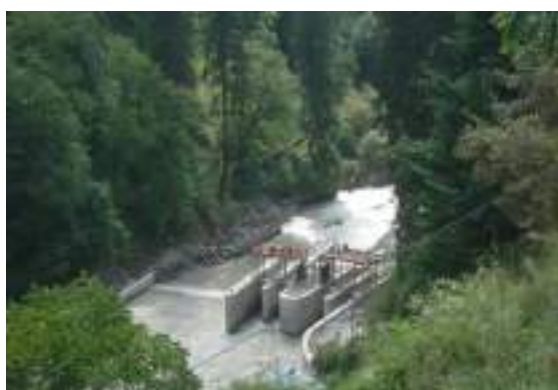
Diversion structure of Balaragha HEP
