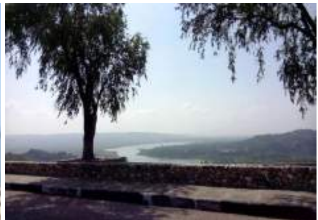
Pong Dam downstream view
