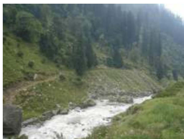
River bank stabilization in Malana Nala
