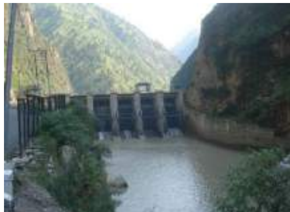
Dam structure of Larji HEP
