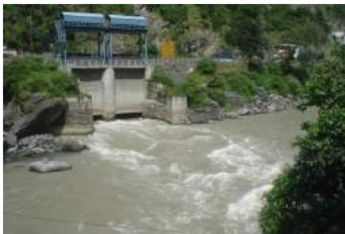
Outlet of Power House of Larji HEP
