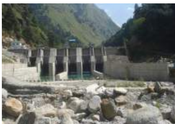
Dam Site of Sainj HEP
