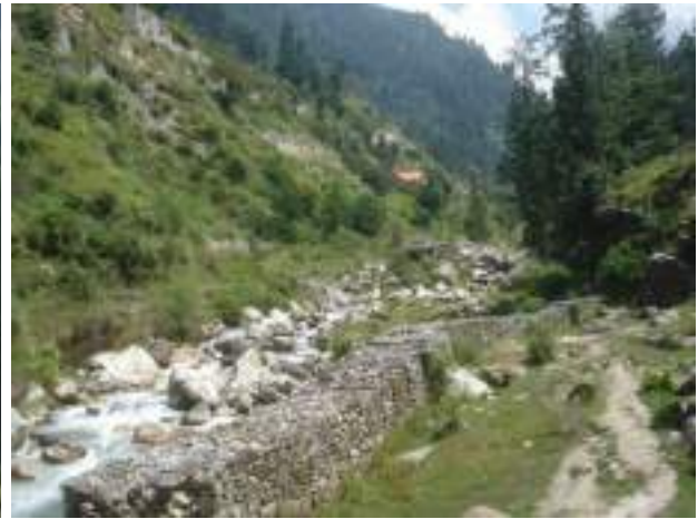
Check walls near river bank of Allain nala
