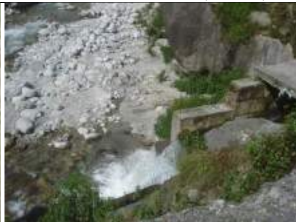
Outlet of power house at Baner Khad
