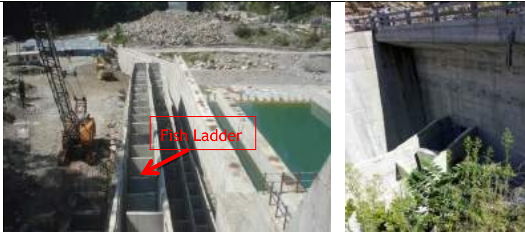
Fish Ladder in Dam structure of Sainj HEP
