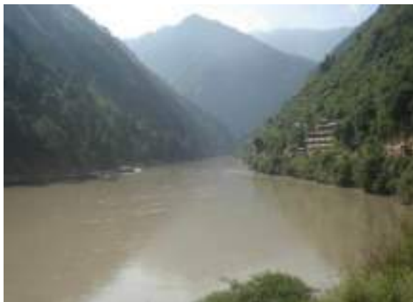
A view of reservoir of Larji HEP
