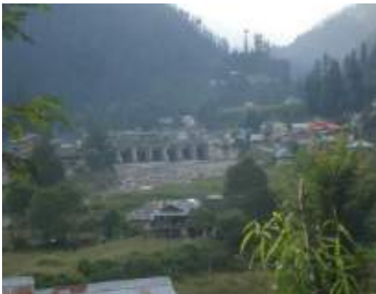
Diversion site of Uhl I HEP
