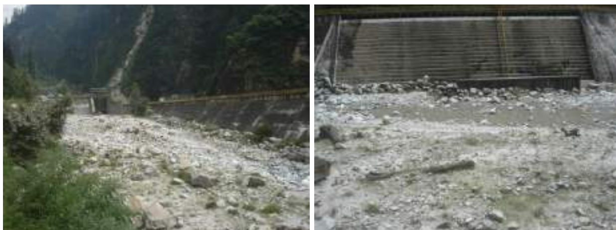
Dry stretch of between diversion and power house site of Malana I HEP
