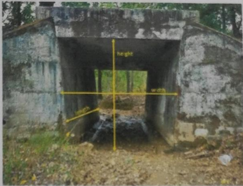
Fig.2 : Dimensions of an underpass determining its openness ratio
