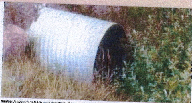
Figure 4 Pipe Culvert
