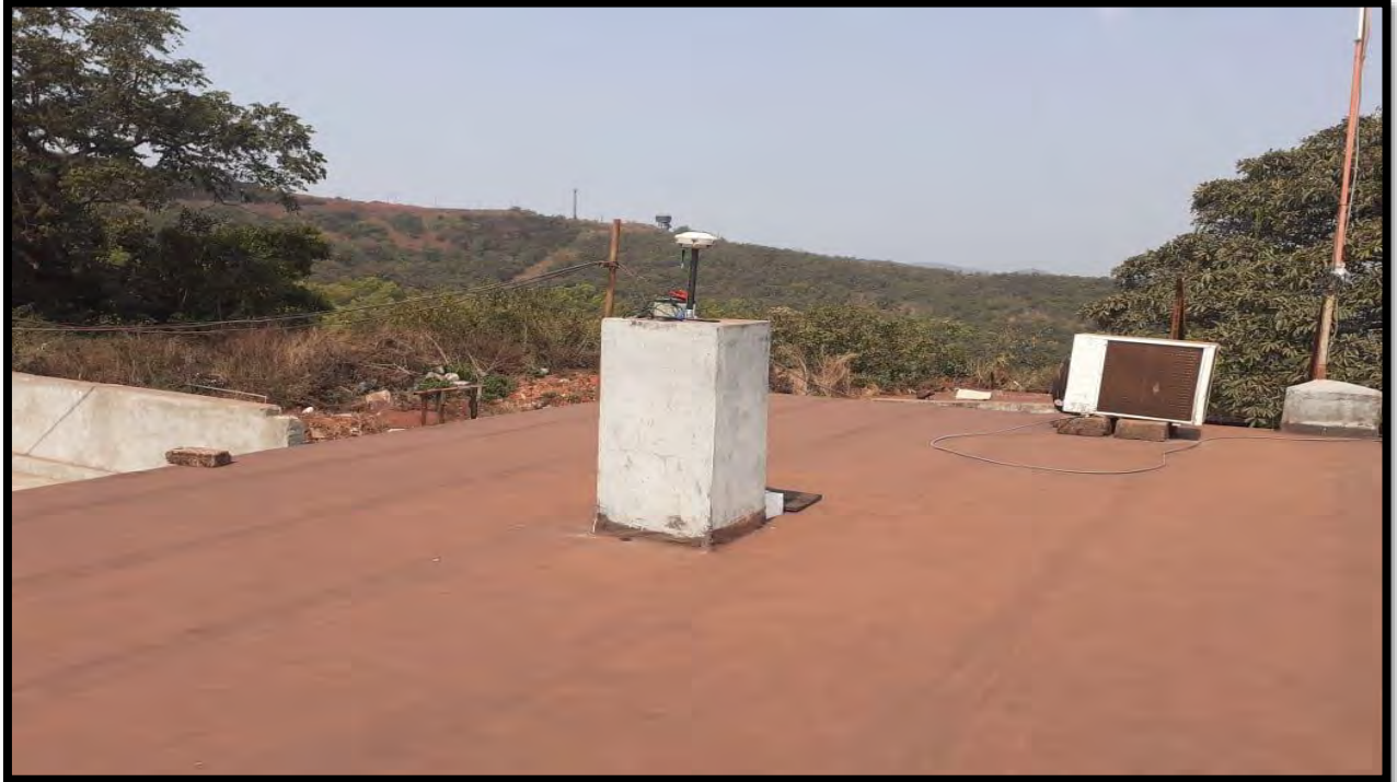
Fig-1: Photo showing Primary Control Point (PCP) Deposit – 5 survey office.
