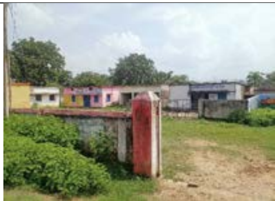
School building in surveyed villages
