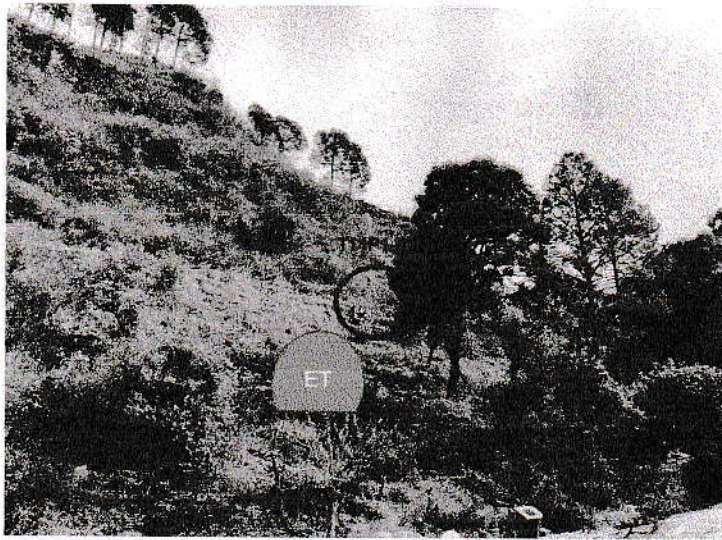
Figure 3 General View of the T-14 P1 (Escape Portal)
