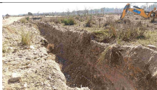
Fig.4 The trench section showing poorly sorted River Borne Material (RBM)
