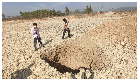
Fig. 6 Section measurement under progress
