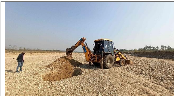
Fig.1 Trenching under progress
