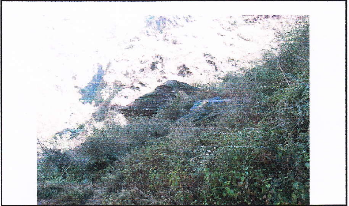
View Showing Dumping Zoone Km 2. (1/6-1/10)
