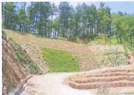
Slope Protection using Bio engineering techniques
