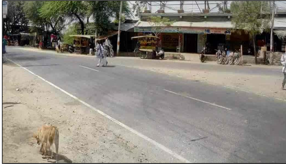
Photo -: End point of the project road
