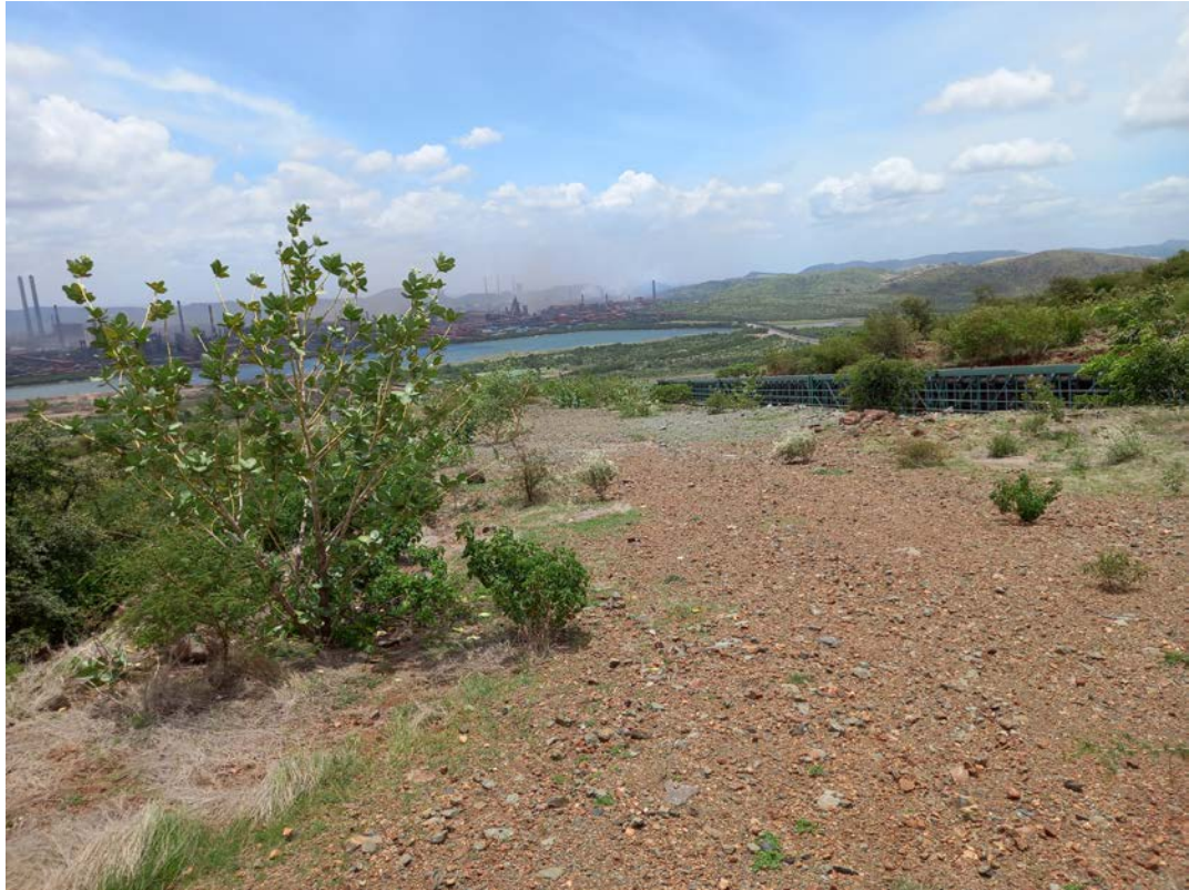
Photograph 1-1 View of NSL of Upper Reservoir
