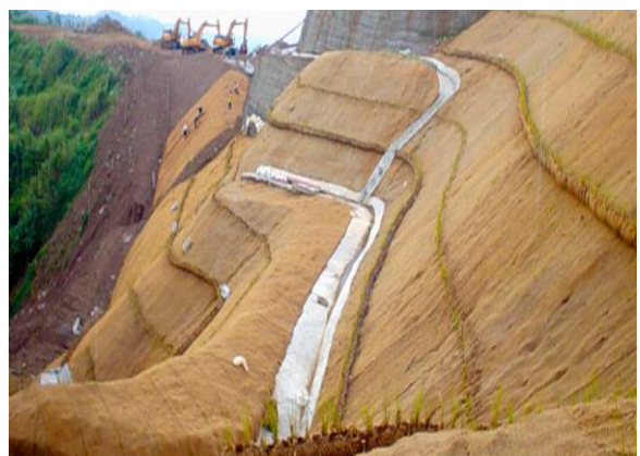
Use of Geo-mats for Slope Stabilization
