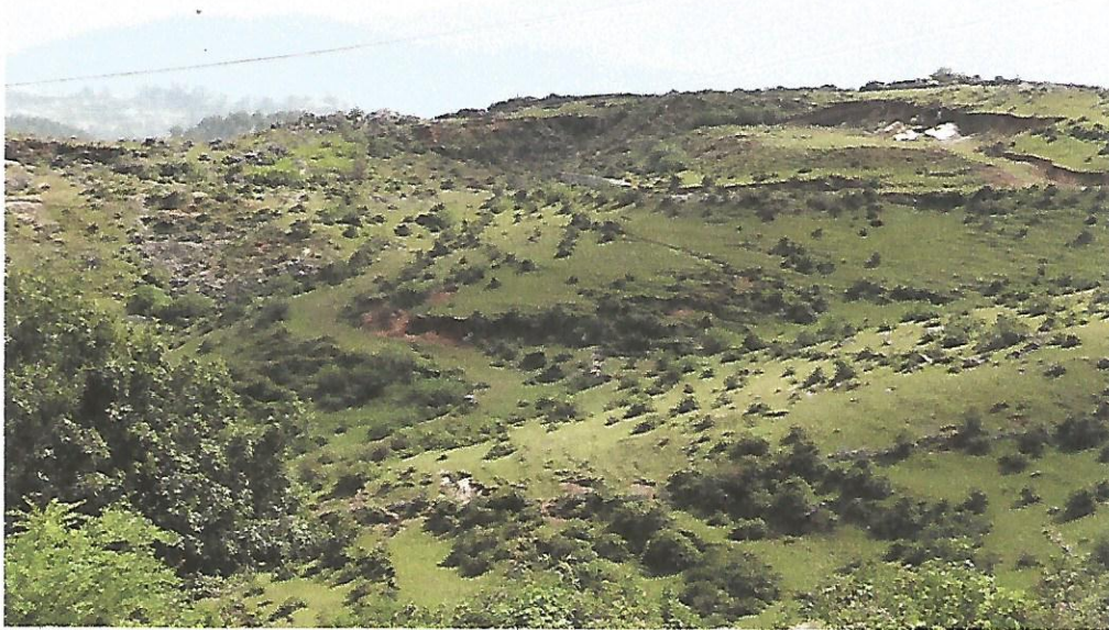
MUCK DISPOSAL POINT NO. 3 KM 2
