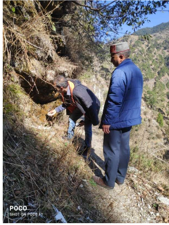
Fig. 2 Weathered gauge material in the joints.
