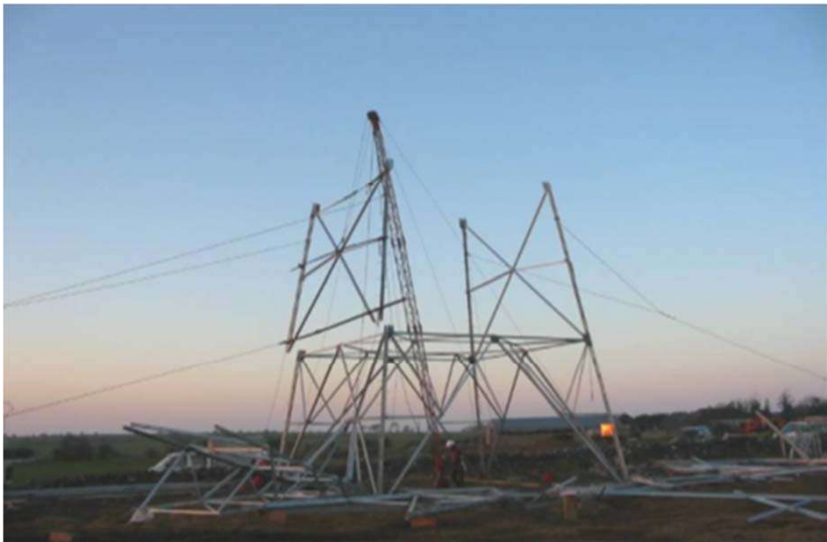
Figure 2.4 Model visual: Derrick pole at tower base
