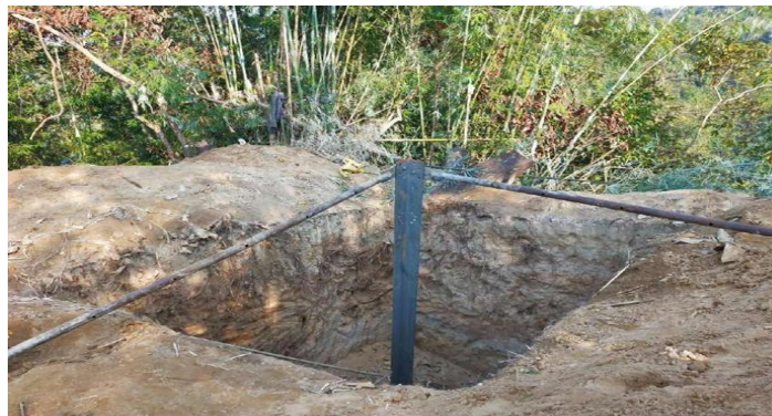
Figure 2.1: Photograph setting template being prepared for final concreting
