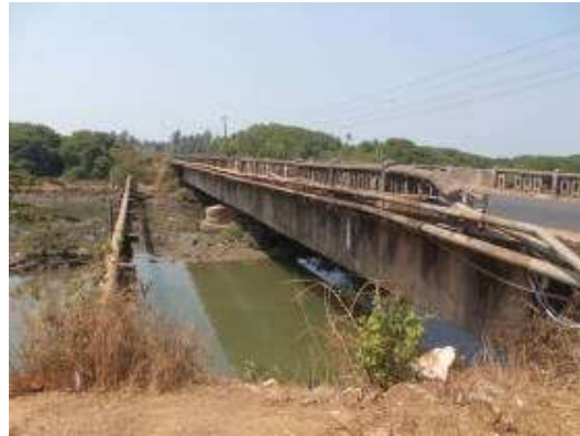
Major Bridge at km 177.600
