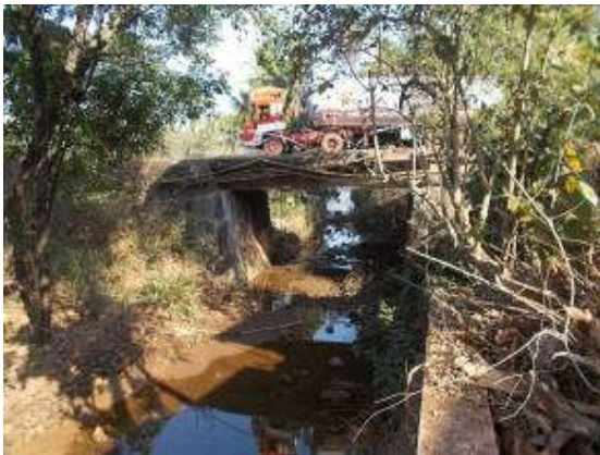
Minor Bridge at km 172.840
