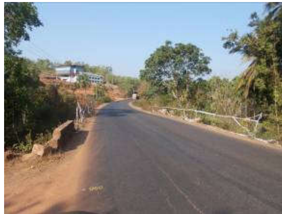
Minor Bridge at km 172.840
