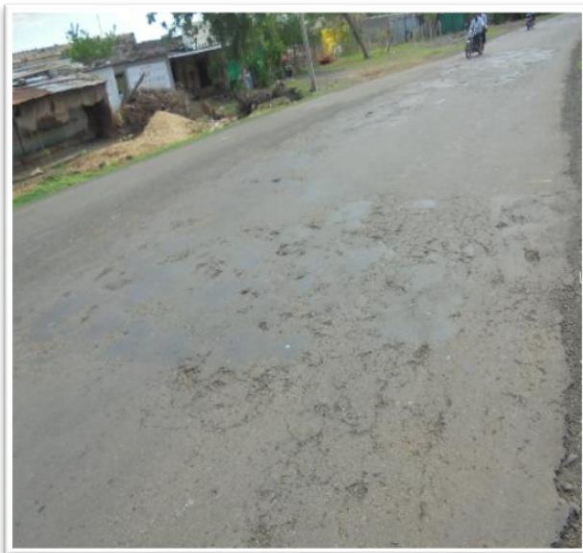
Photo 3:- Map Cracking
