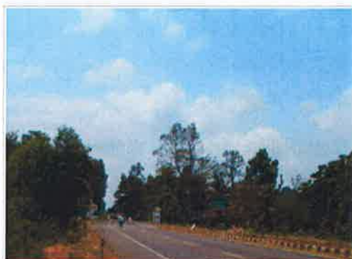
Fig. 1.1: Starting Point of the Project
