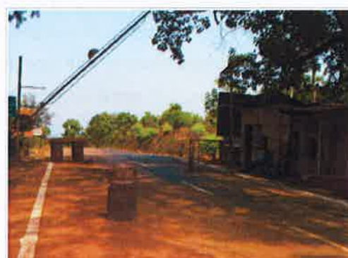
Fig. 1.2: End of the Project Stretch
